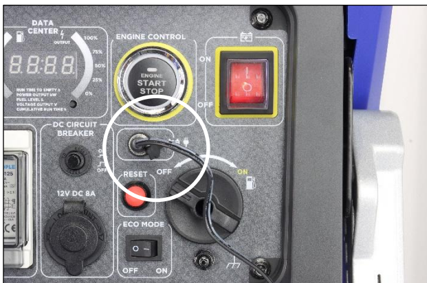
Figure 17 Connect the Battery Charger to the Generator
