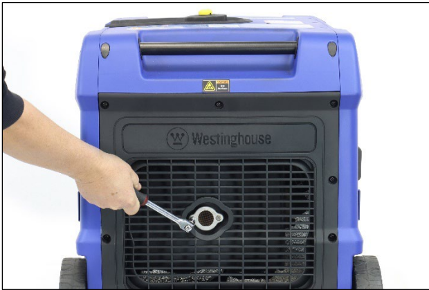
Figure 46 Remove the Spark Arrestor Clamp
